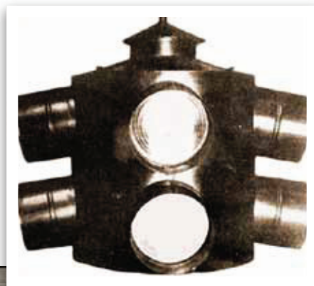
▼ An example of the first electric traffic signal developed by Lester Wire in Salt Lake City, Utah, 1912.
